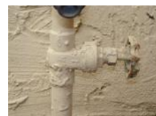
Old gate valve
